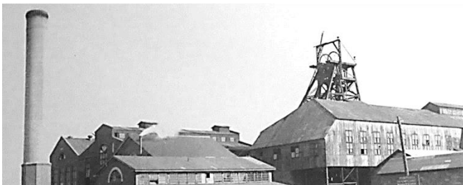
Allan Shaft, Stellarton, N.S. Coal Mine where both Elaine's father and grandfather worked. Picture ca 1930's
